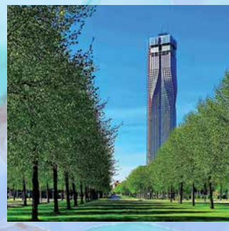
Karlatornet - at 246m Scandinavia's tallest building and probably its most elegant too. Pic by Skyscraper City
