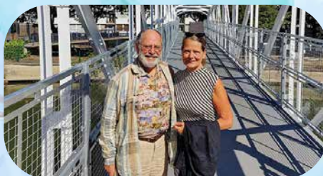
Marie and Ralph on the renovated and repainted pedestrian bridge close to our house. After a couple of years it was opened for a few weeks then closed again for further work.
