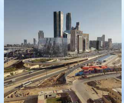
View of part of the financial district from my hotel window. There were vast areas of cleared land and forests of cranes everywhere in the City.
