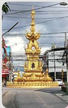
Chiang Rai's splendid clock-tower behind a maze of cables
