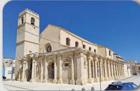
The church of St Lucy, built on the site of her alleged martyrdom in the fourth century. The great glory of this building is its Caravaggio - The Burial of St Lucy
